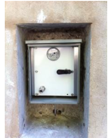
Ground Level fill-in-place
